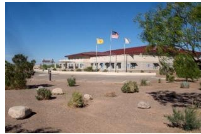
Brackish Groundwater National Desalination Research Facility Alamogordo, NM
