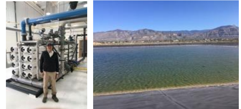
Alamogordo 1MGD Desal Plant
