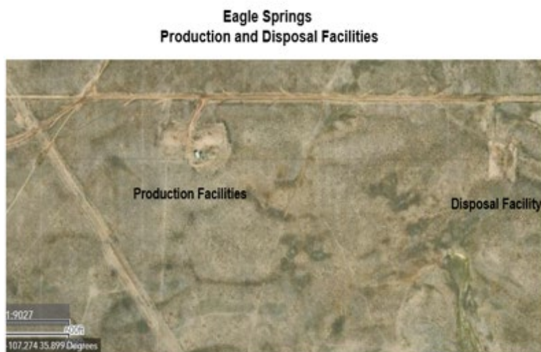
Figure 2. Eagle Springs production and disposal facilities.
