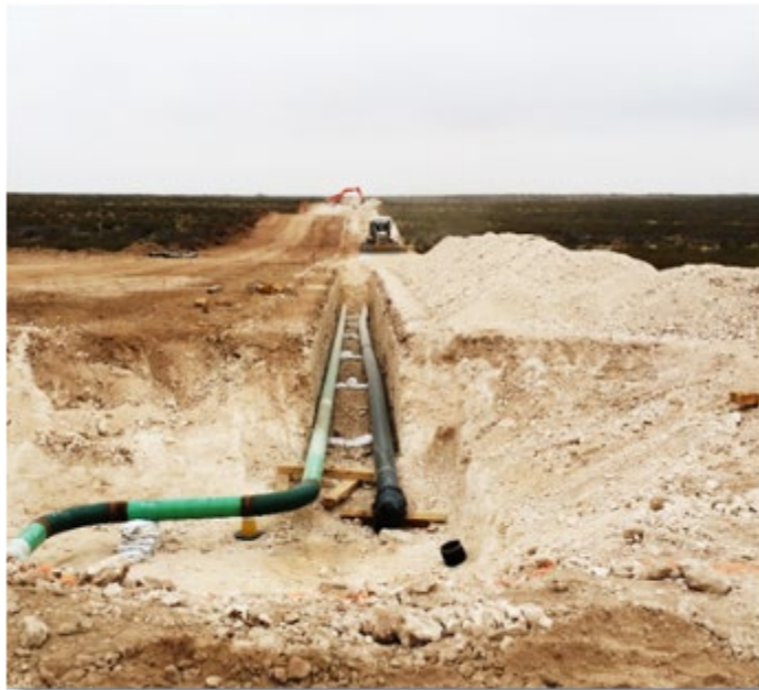
Figure 2-A-3: Water and oil pipelines being jointly constructed in the Delaware Basin.
