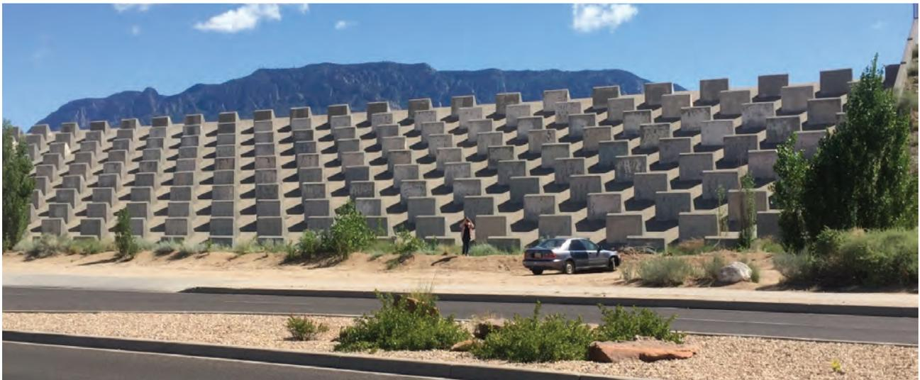
**Figure 8.7.** Photo of the emergency spillway for the John Robert dam owned by the Albuquerque Metropolitan Arroyo Flood Control Authority (AMAFCA). The spillway was designed to convey a flow of 23,600 cfs from a PMP storm. *Photo by Bruce M. Thomson*
